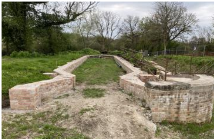
Dry-dock walls restored. Under the safety of the grass, brick floor with pitch/tar evidence of boat repairs. Credit: Howard Wilson
