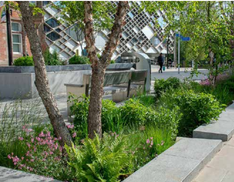
Figure 53: Raingardens with outlet kerb in stone
