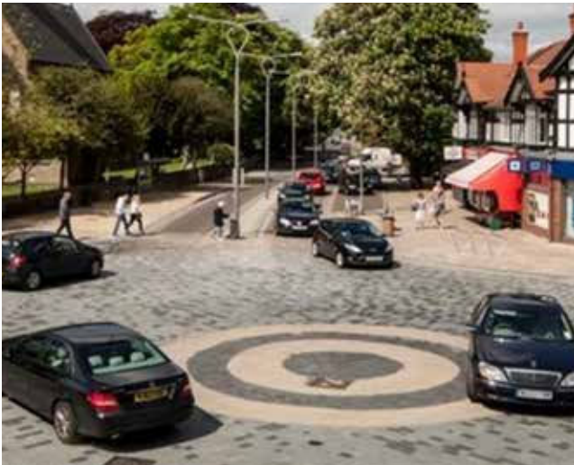
Figure 67: Distinctive materials for junction, footpath, use of shared surface for all users to reduce traffic speed in Poynton
