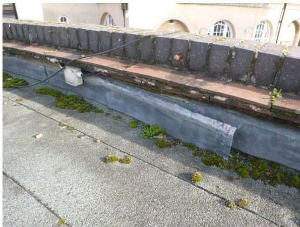
Lead flashings to the parapet upstands
