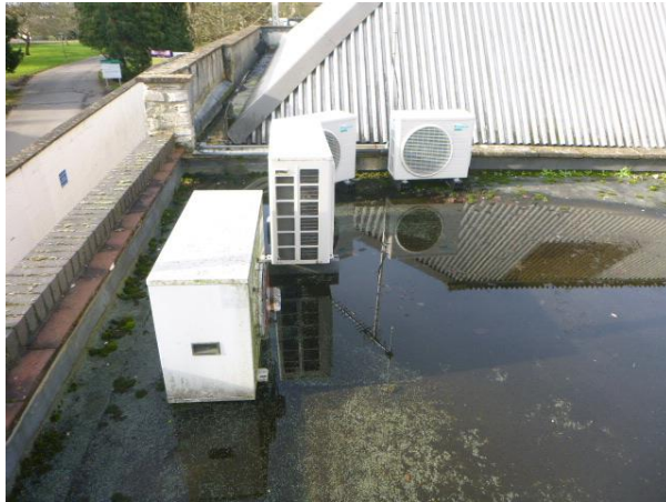
Gradient on flat roof
