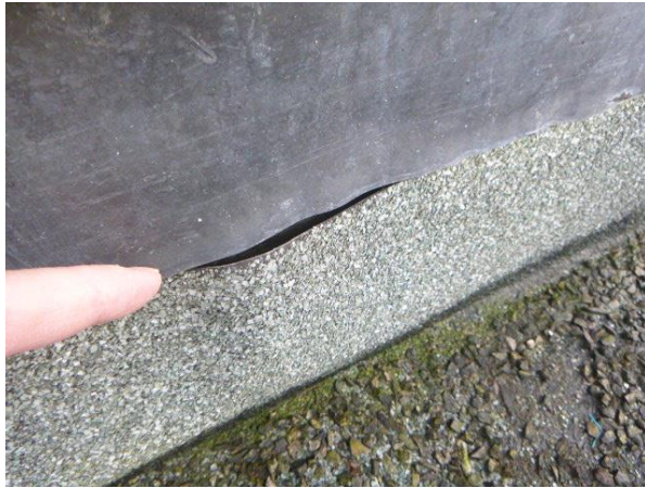
Flat roof felt upstand and lead flashing
