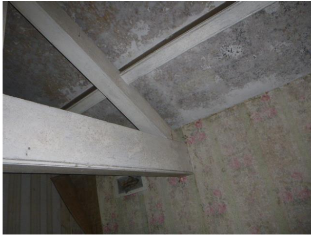
King post trusses embedded in the solid wall of the older section of the central core
