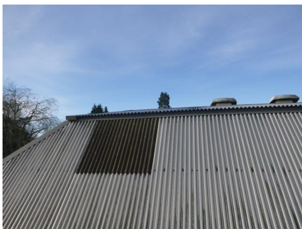
GRP roof light to the metal clad roof
