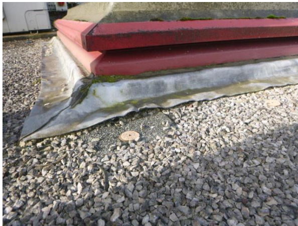
Lead upstands to office/foyer rooflights
