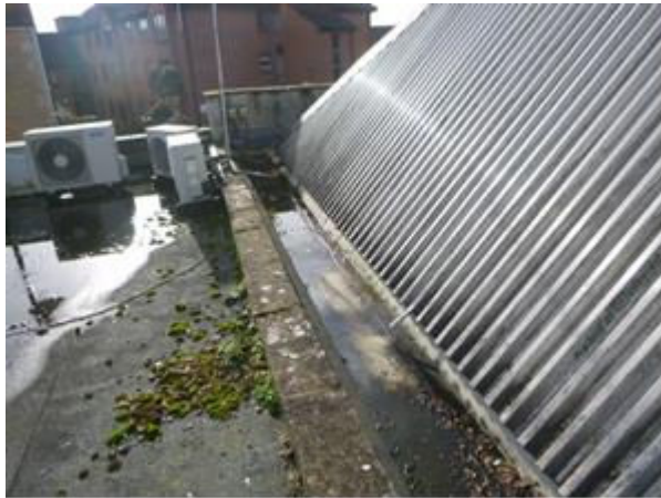
Metal pitched roof, parapet gutter, and copings
