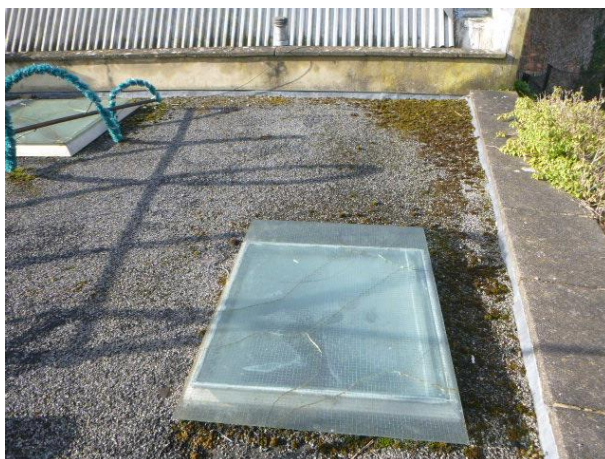
Cracked Georgian wired roof lights over the Dressing Rooms.
