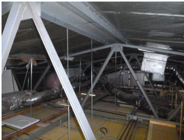
View across the Assembly Hall roof void steel trusses
