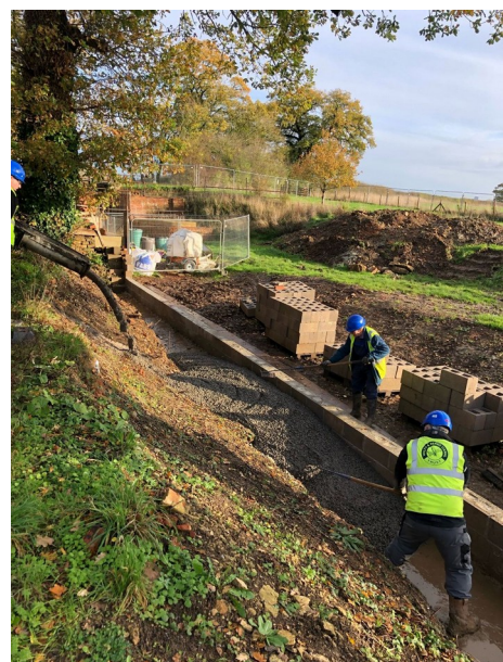
WaitingWall: back-filling with concrete
