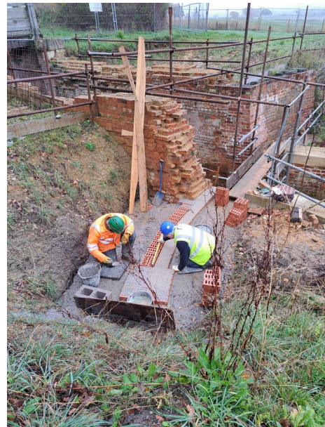
bull-nose walls at Top Lock taking shape
