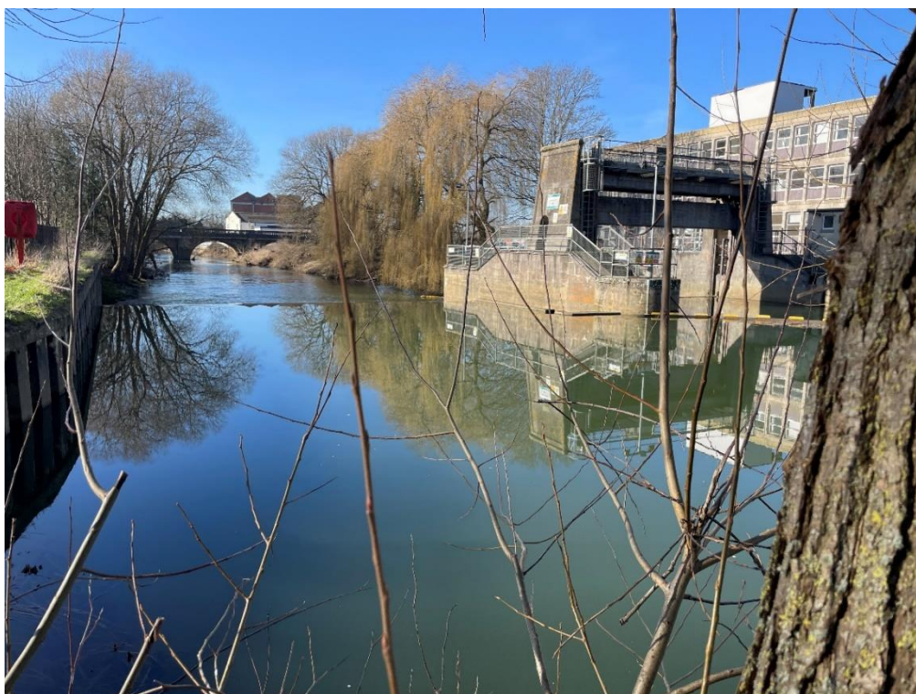
Figure 8. Upstream of Melksham Gate, looking downstream at the weir (left), fish pass (middle) and sluice gate (right). The bank to the left is a sheet-piled wall with concrete capping.
