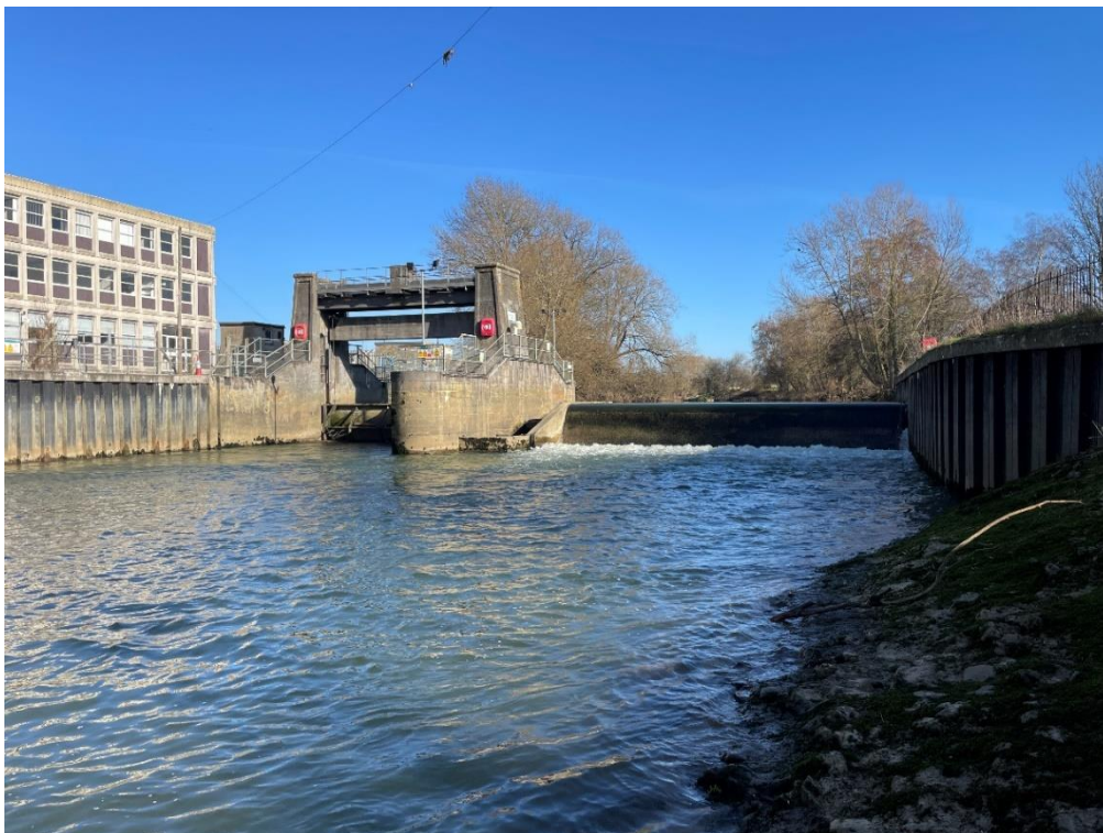
Figure 7. Downstream of Melksham Gate looking upstream at the sluice gate (left), fish pass and weir (right). The bank to the right is a sheet-piled wall with concrete capping.
