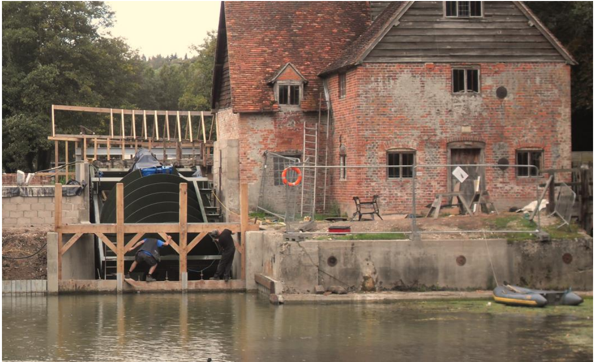
Figure 15. Example Archimedean Screw turbine during construction. The screw is a 3.6m diameter screw, spanning a head of 1.8m and discharging 7.8 m 3 /s. This is almost identical to the screw specified at Melksham Gate.
