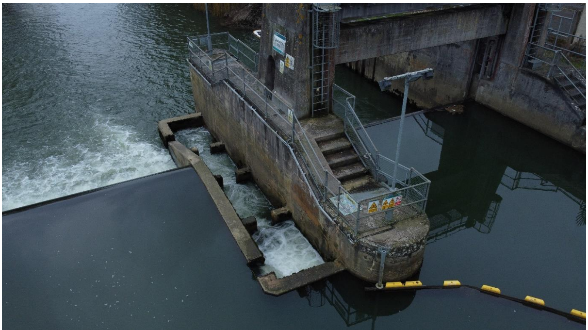
Figure 11. Pool and traverse fish pass located between the weir and sluice gate
