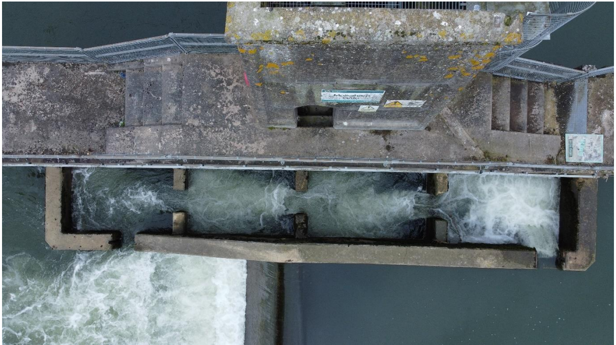
Figure 10. Pool and traverse fish pass located between the weir and sluice gate
