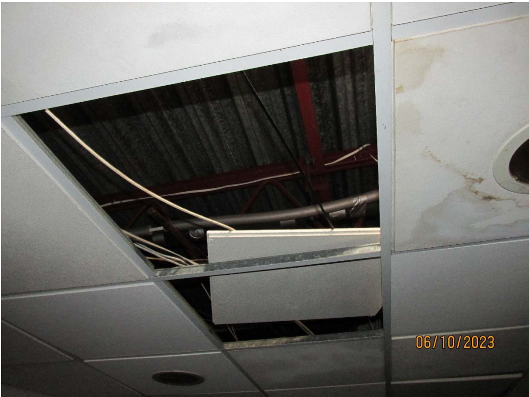
Roof structure above suspended ceiling in Foyer
