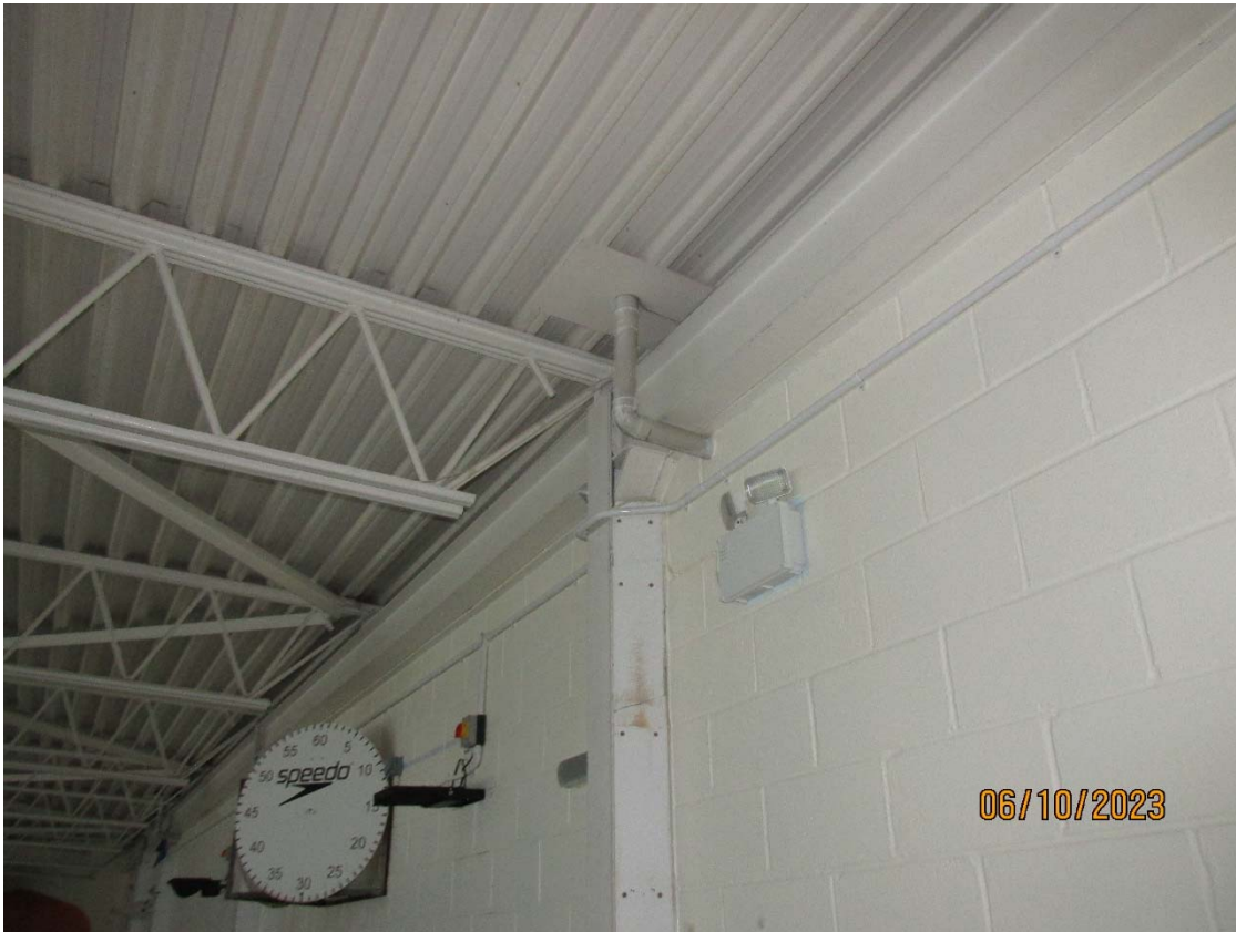
Eaves beam on steel columns supporting Lattice Roof trusses above the Swimming Pool
