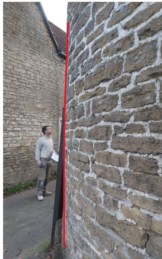
Figure 2 – bowing of wall caused by slumping and sagging of masonry structure
