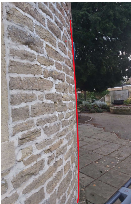
Figure 2 – bowing of wall caused by slumping and sagging of masonry structure
