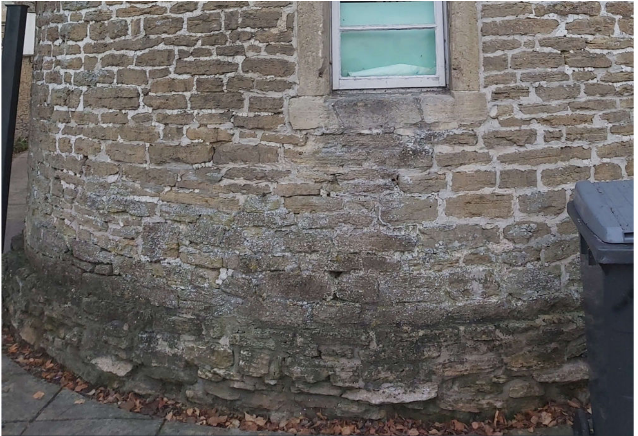
Figure 1 – stone erosion from salt splashback
