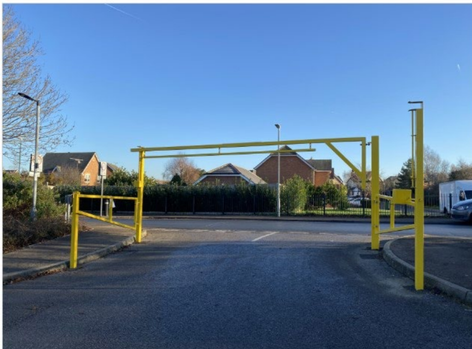
Overhead car park barrier:
